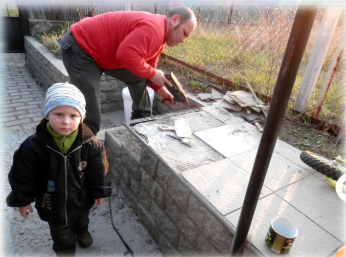
(Essential repairs for our Genesis House)
